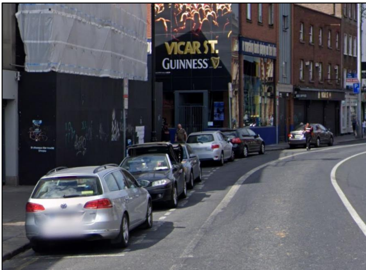
Image 11.2: Commercial Parking Impact – Parking Bays to be Removed
